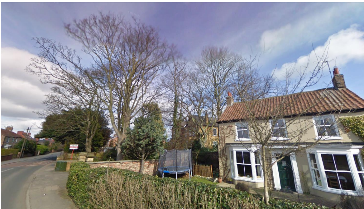
View of frontage October 2022
